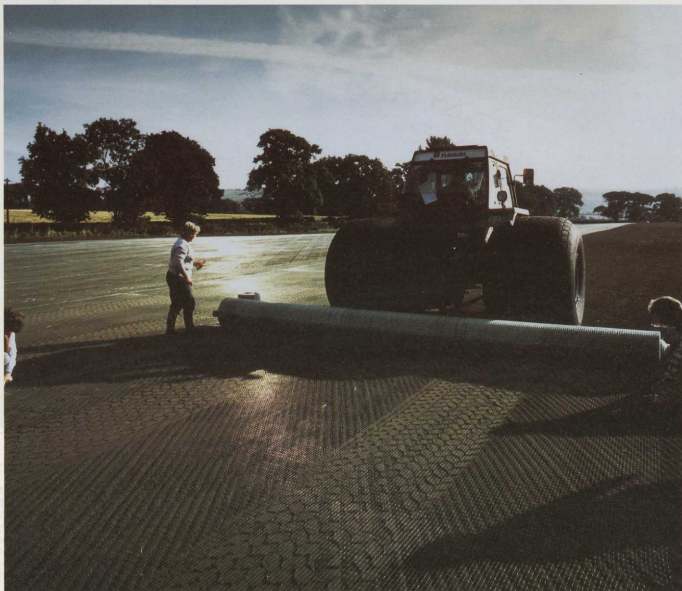
SODNET being laid on Lindum turf fields.
