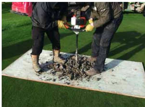
Drilling 1.3 metre hole with powered auger
