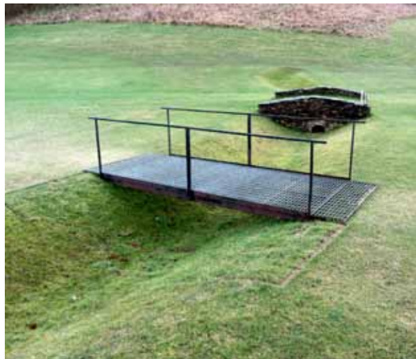
Transportable bridge made by greenkeeping team
