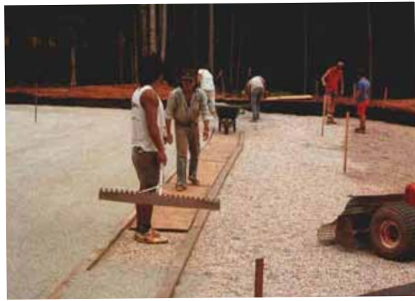
Fig.2: Time consuming installation of a coarse sand intermediate layer (Hummel, 1993)
