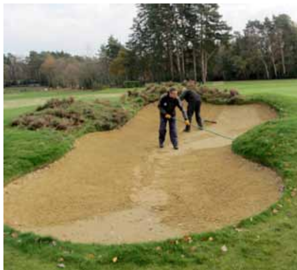
ABOVE TOP: Fairway bunker complete and base consolidated prior to sanding
