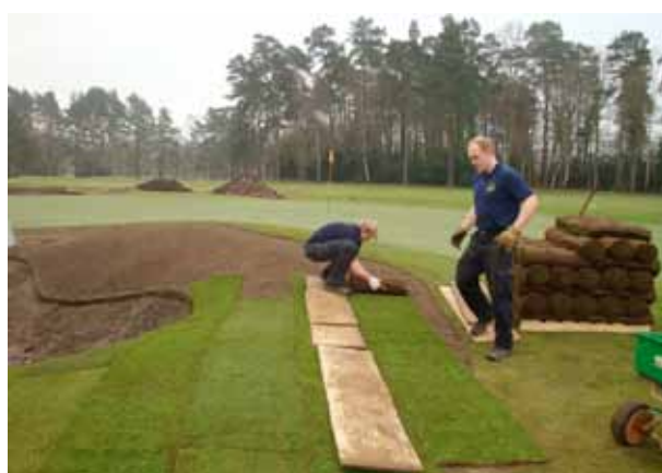
MAIN ABOVE: Greenside bunkers largely completed and ready for turfing
