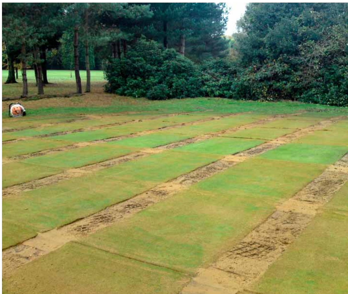
ABOVE: Greens drained via Wizz wheel trencher
