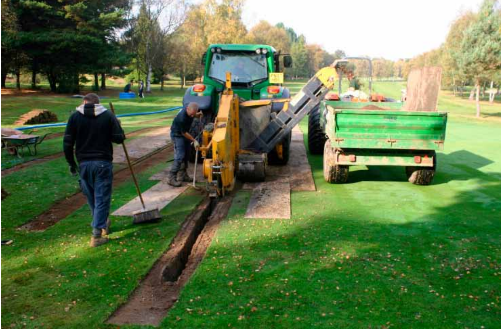
ABOVE: Greens drained via Wizz wheel trencher
