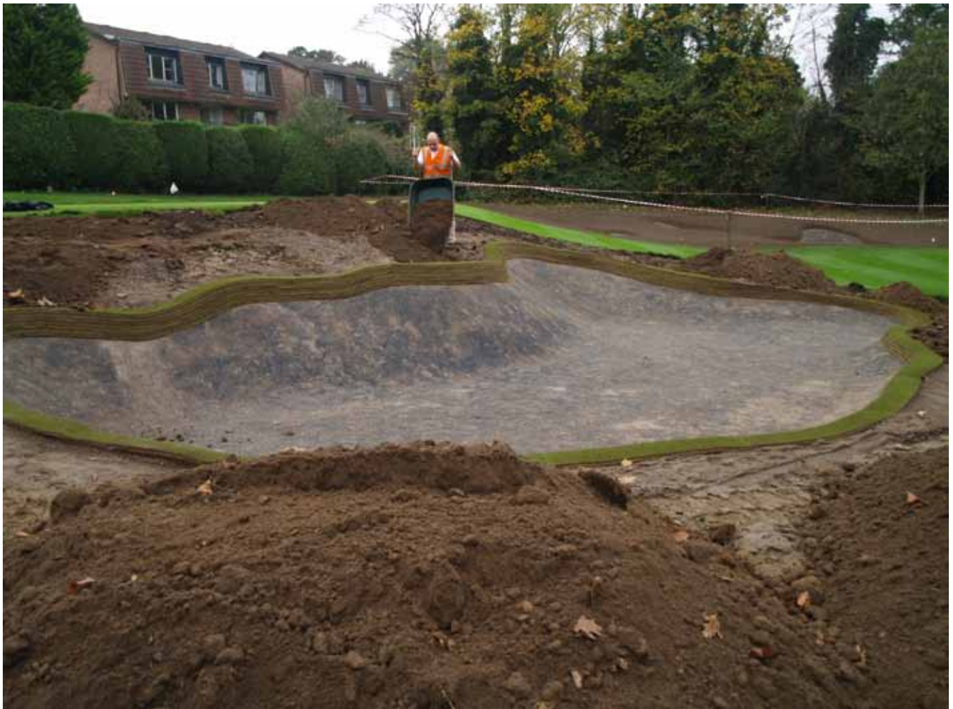
ABOVE: A renovated bunker under construction at Wimbledon Park Golf Club
