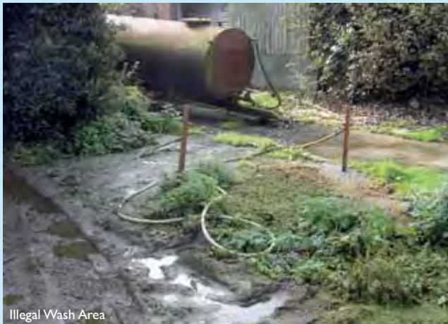
Illegal Wash Area
