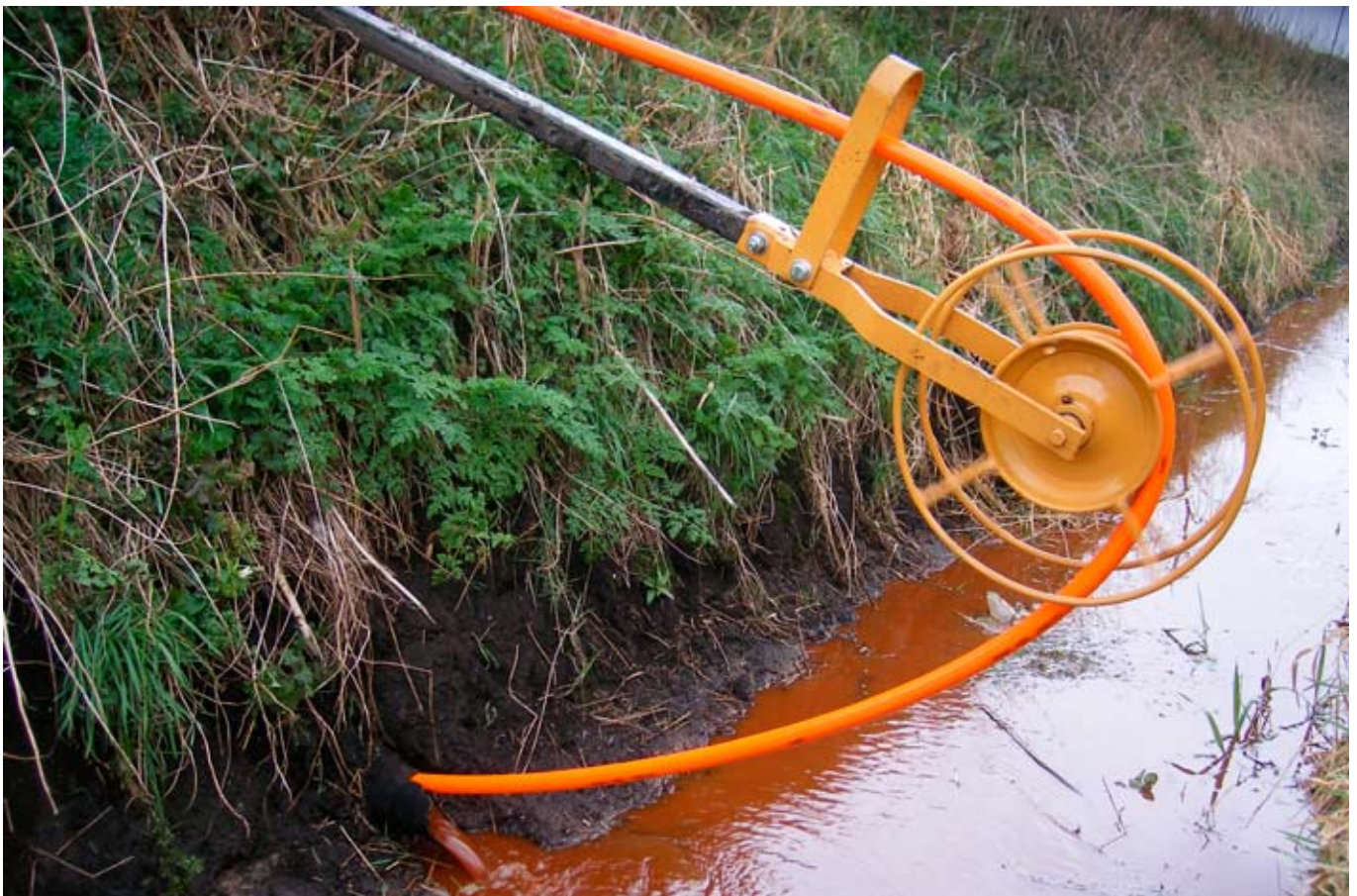
Ochre is a particularly common sediment found in primary drainage systems in certain parts of the country; note the rusty brown deposits flushed from the pipe pictured. Mastenbroek jettors are typically used for agricultural field drains, but there is no reason why they cannot be employed in sports turf drainage.
