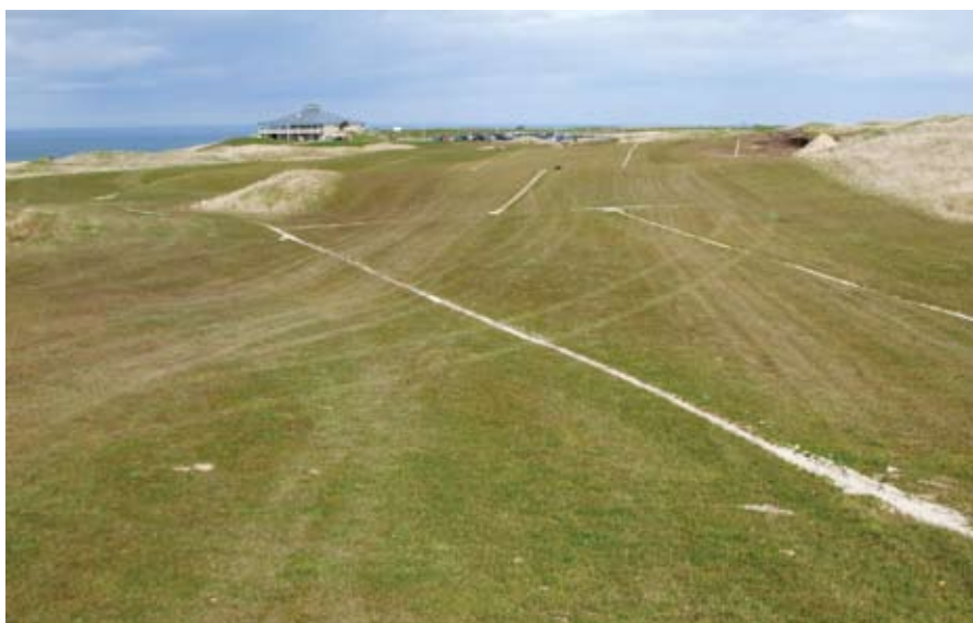
Drainage lines at Fairmont St Andrews - Copyright MJ Abbott Limited
