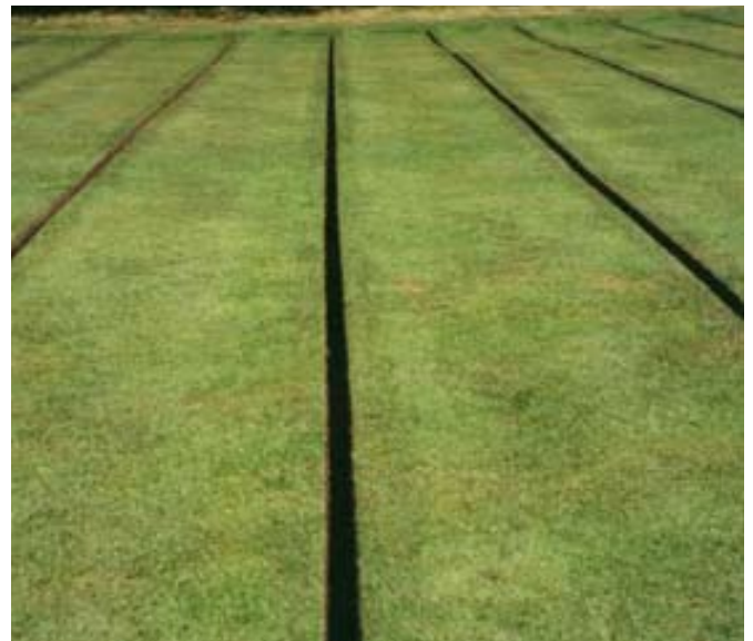
Neat clean trenching
