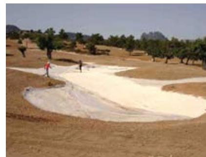
Covering bunkers with plastic
