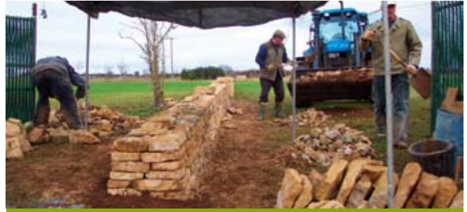
Large stones are put into the foundation and base courses, followed by progressively thinner stones for the uppermost courses.
