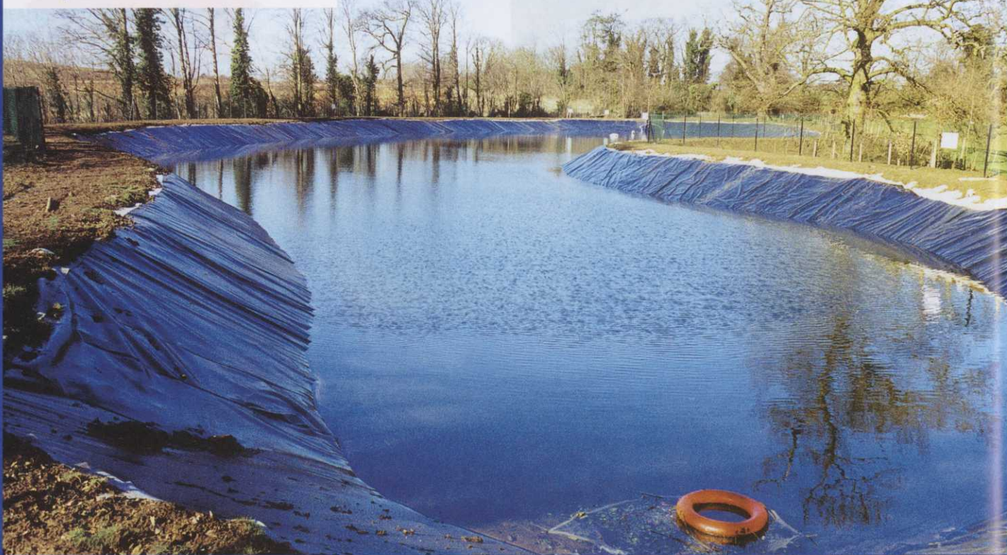
Hanbury Manor Golf Club: Reservoir Liner
