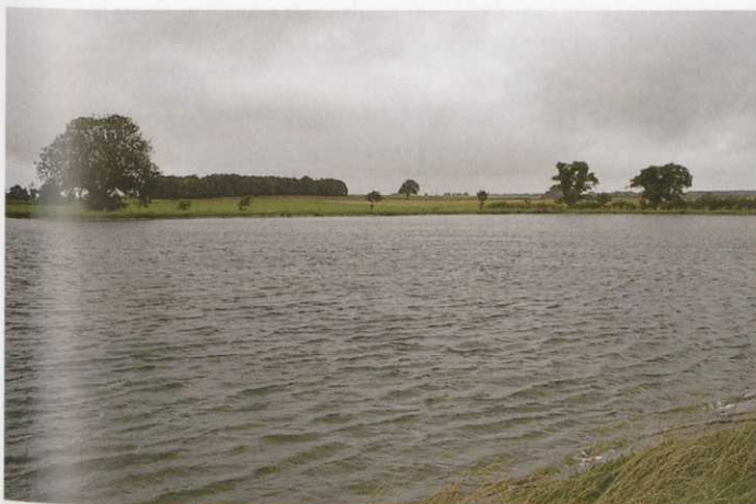
42,000m 3 synthetically lined reservoir
