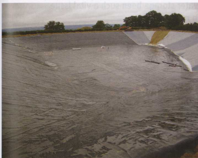
A lined reservoir not far off being ready for filling
