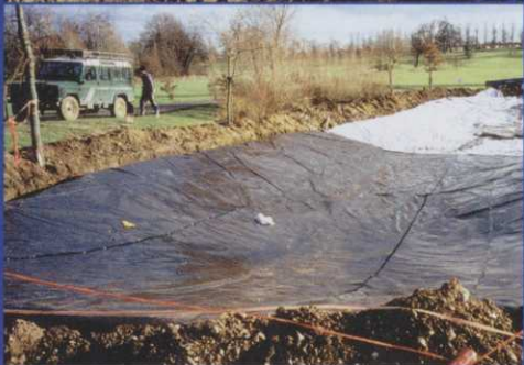
Donnington Grove Golf Club: Pond Liner
