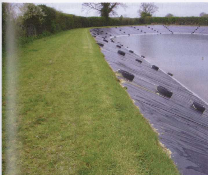
Finished embankment surface
