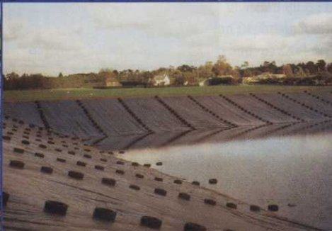
Frilford Golf Club: Irrigation Reservoir Liner
