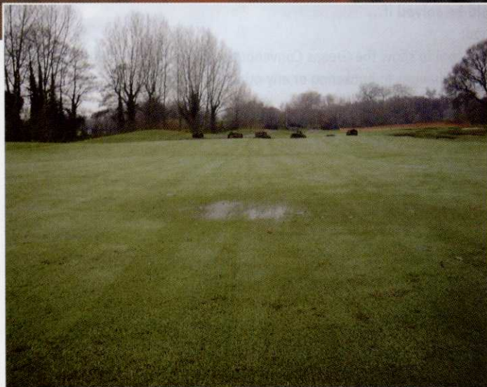
Standing water on fairway
