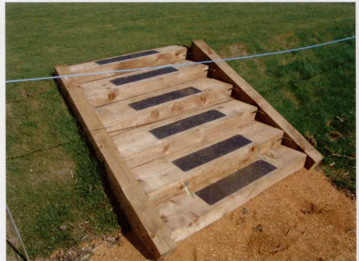
The team do all construction work in-house
