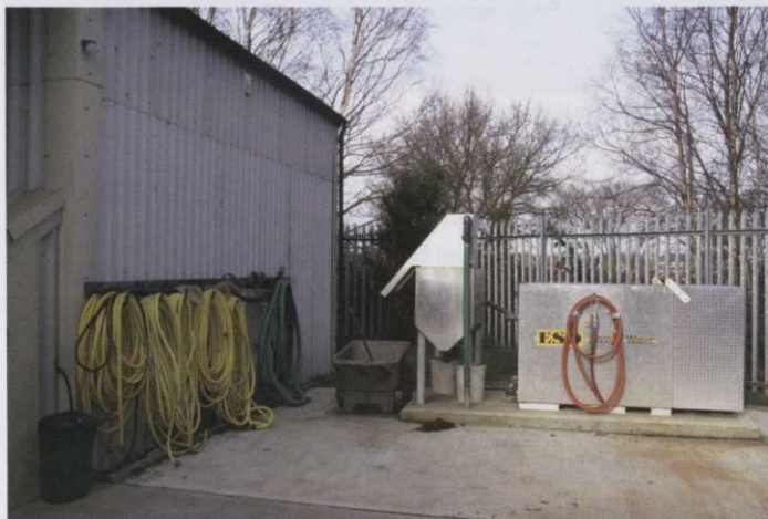
It may well take time to recoup the cost of a washing water recycling plant, but such a system demonstrates environmental awareness. This can help when it comes to negotiating irrigation water supplies, particularly in a dry year
