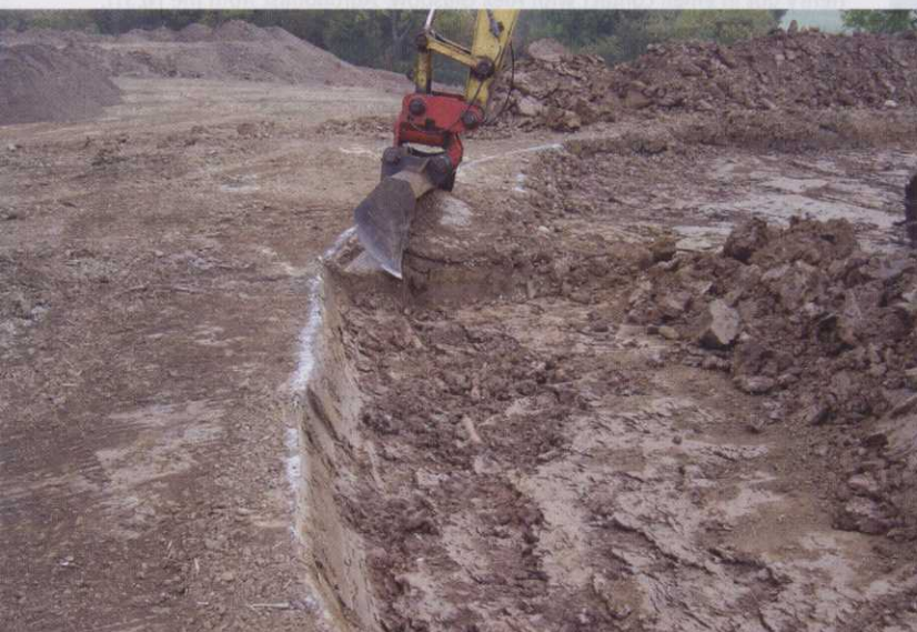
▲ Digging out the pit in ideal conditions
