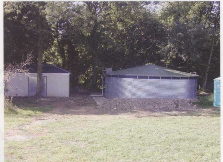
The state of the art irrigation system installed at Bath Golf Club will reduce water usage dramatically
