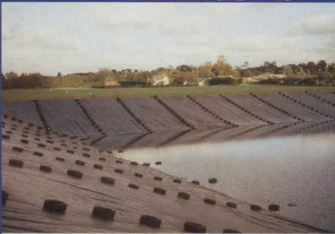
Frilford Golf Club: Irrigation Reservoir Liner
