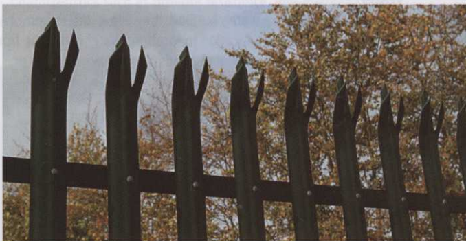
The tops of security fencing posts come in a range of style, this one is called the trident.
