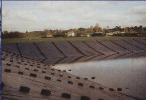
Frilford Golf Club: Irrigation Reservoir Liner
