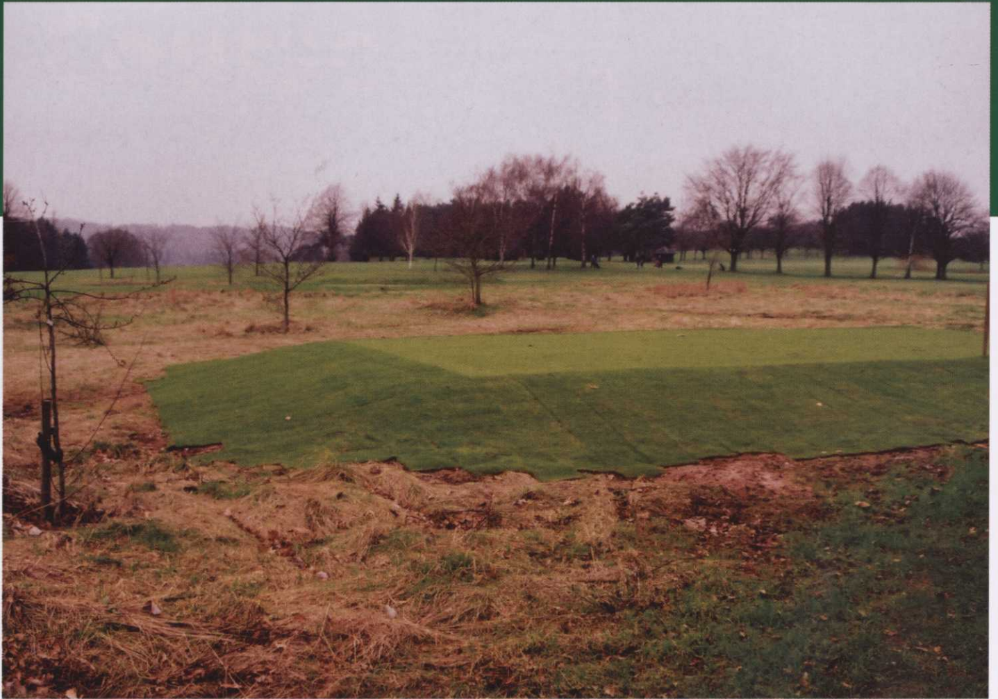
▲ A new tee built over the winter
