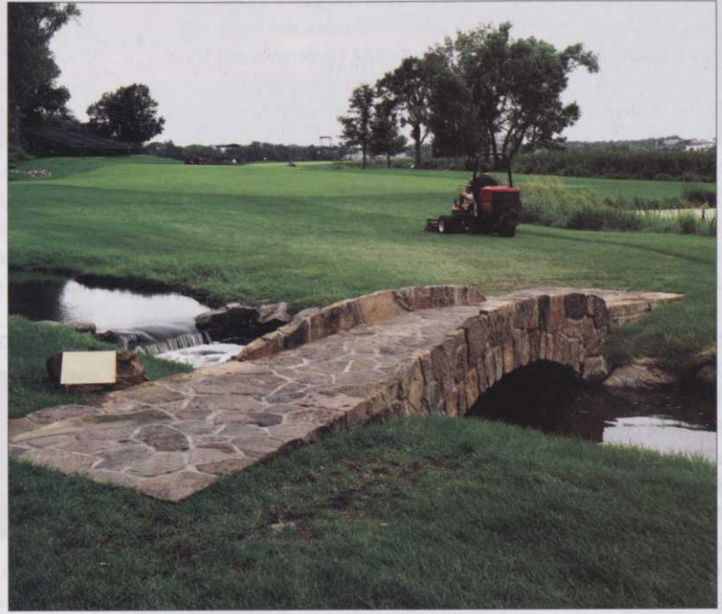
▲ A finely built stone bridge
