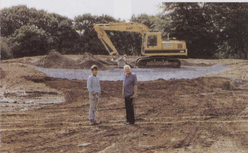
Author Jim Arthur (right) oversees the spreading of root zone over a blinding layer of Cornish grit.
