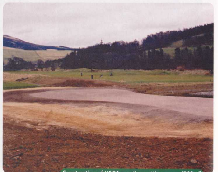
Construction of USGA practice putting green (800m 2 )
