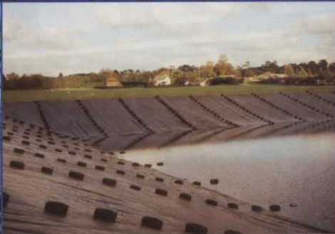
Frilford Golf Club: Irrigation Reservoir Liner
