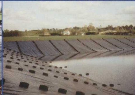
Frilford Golf Club: Irrigation Reservoir Liner
