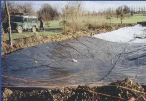
Donnington Grove Golf Club: Pond Liner
