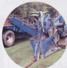
20 Pinpointing Drainage Needs
