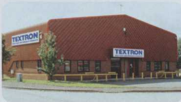
The hub of the Yorkshire operation is the 8,500 square feet modern premises at Selby. This depot also has 18,000 square feet of secure outside storage.
