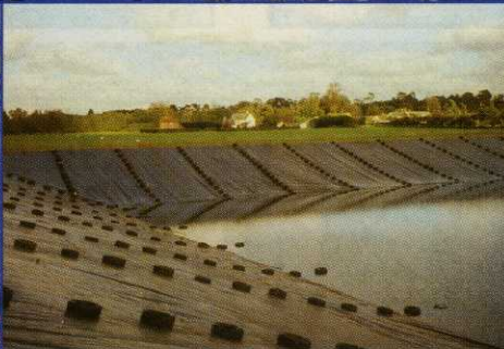
Frilford Golf Club: Irrigation Reservoir Liner
