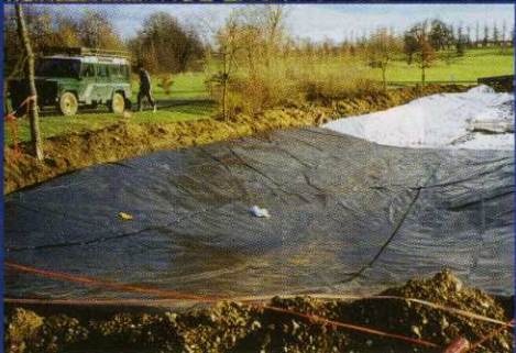
Donnington Grove Golf Club: Pond Liner
