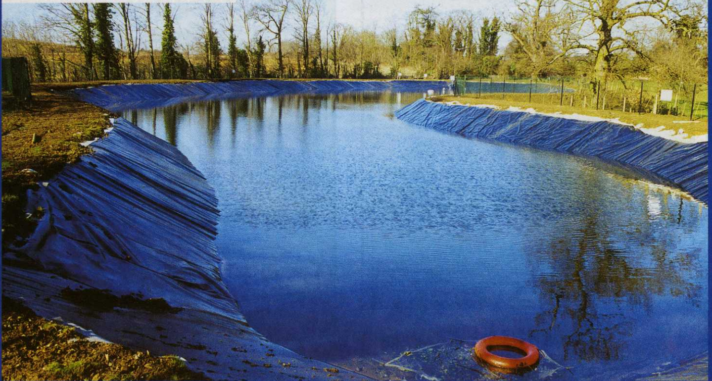
Hanbury Manor Golf Club: Reservoir Liner
