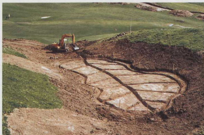
The new 18th green showing herring-bone and perimeter drain lines
