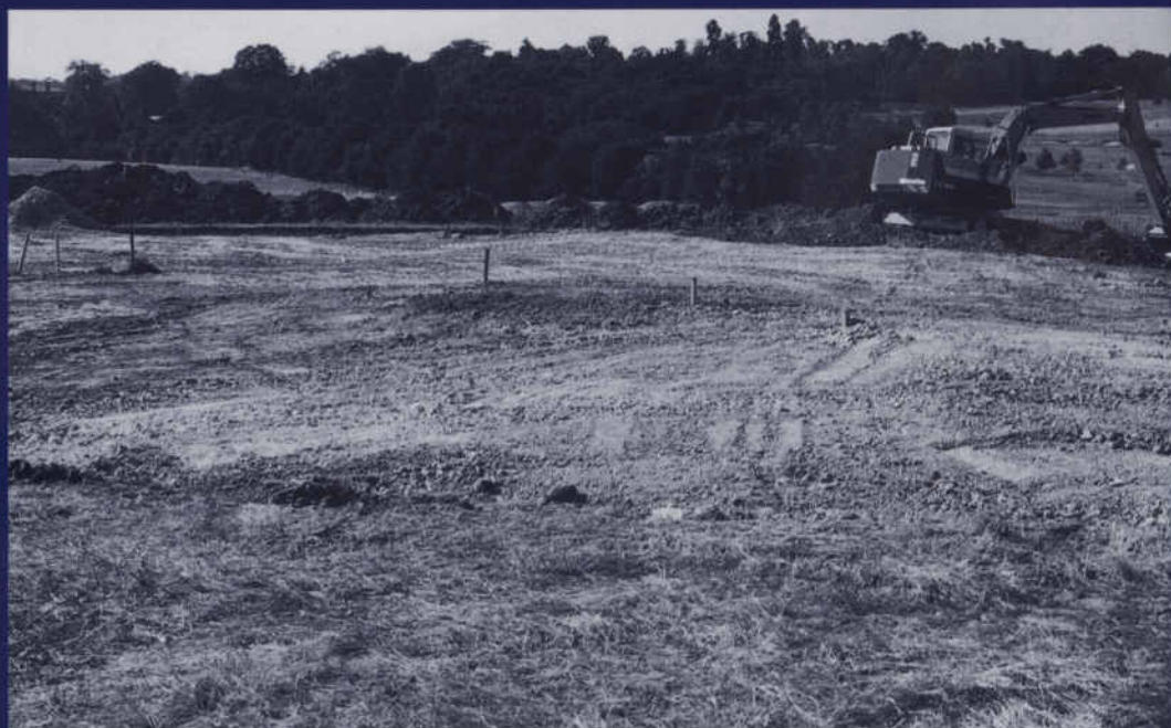
Below: Rochester and Cobham Park during reconstruction
