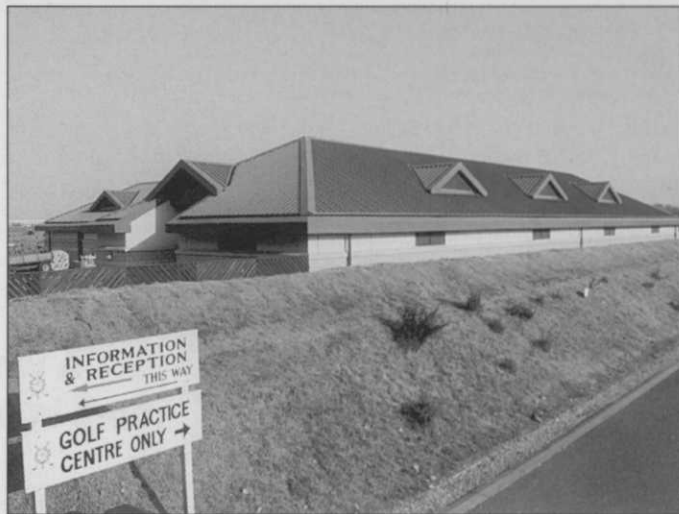
A 2m high embankment around the facility provides an effective and economical screen. Air circulating through ducts beneath the eaves and in the roof provide five air changes an hour within the building
