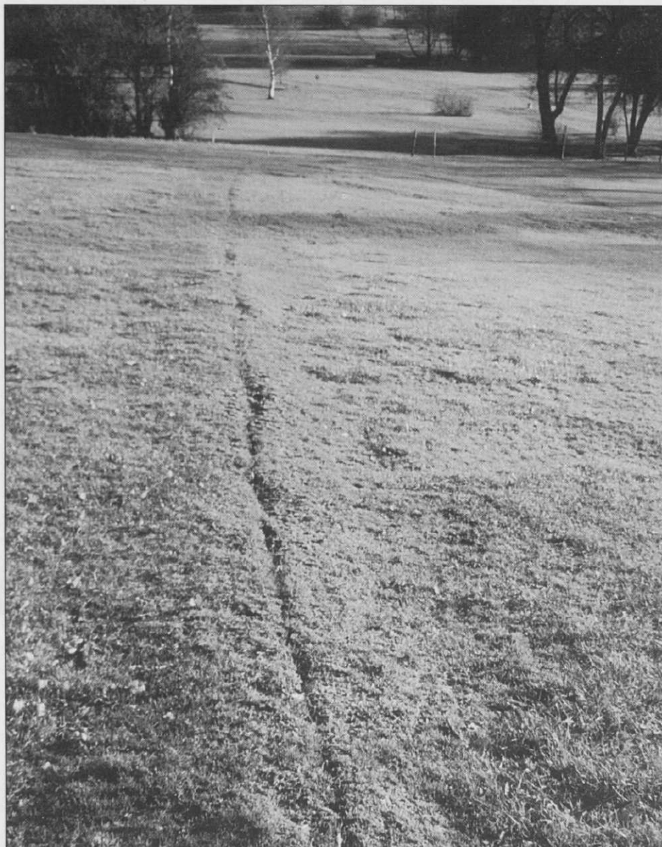
Now you can hardly see the join: After the work the heave has gone and the fairway is returning to normal
