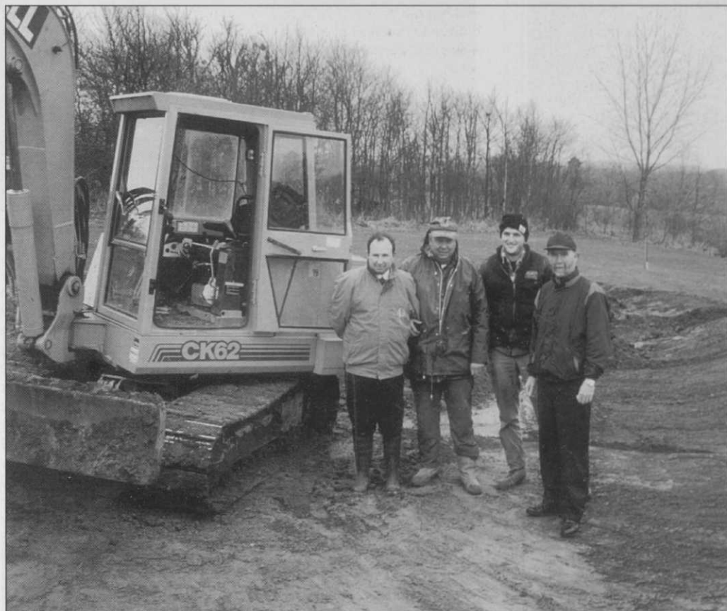
Ian Scott Taylor, left, and Bill Sparrow, right, with two members of Cousell Associates Ltd construction team
