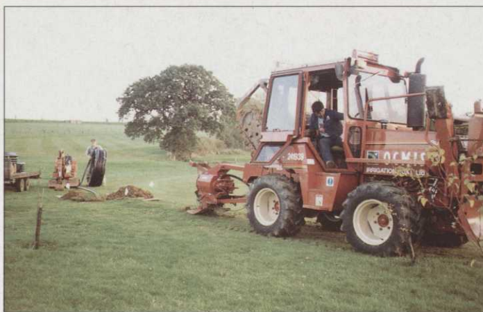
The Ocmis installation team in action. Far left, late evening irrigation
