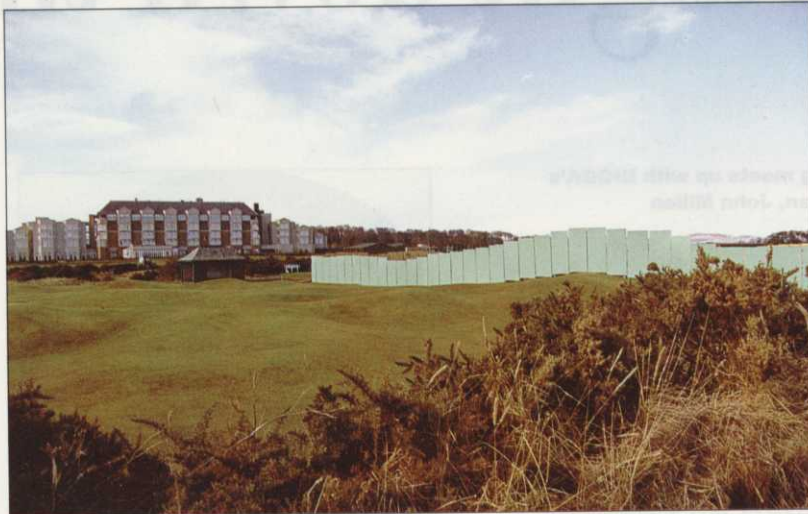
Screens hide the work underway on the new £3m clubhouse
