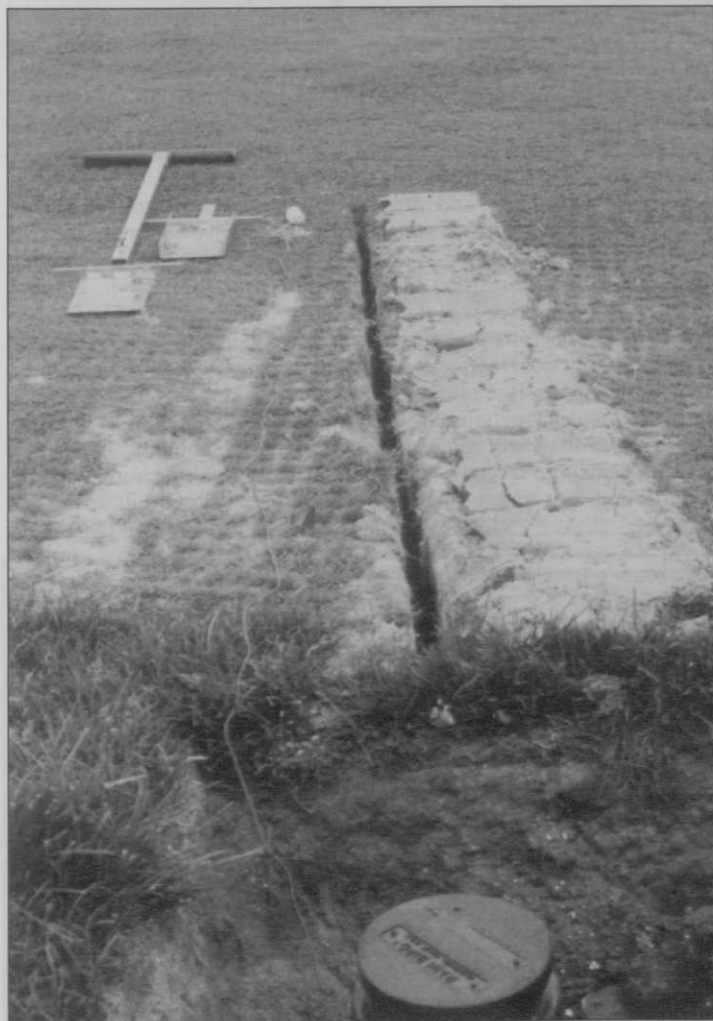
Installed: a moisture core in the green
