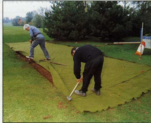
Erosion problems at Sceptoft Golf Club. The pictures show the appalling state of a high wear area and VHAF carpet being installed below the surface, through which natural grass will grow. Photographs courtesy of Notts Turf
