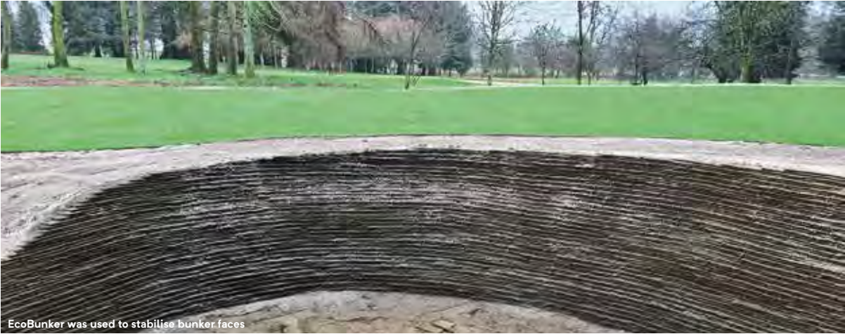
EcoBunker was used to stabilise bunker faces
