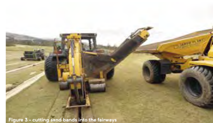
Figure 3 - cutting sand bands into the fairways
