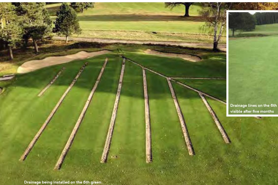
Drainage being installed on the 6th green
