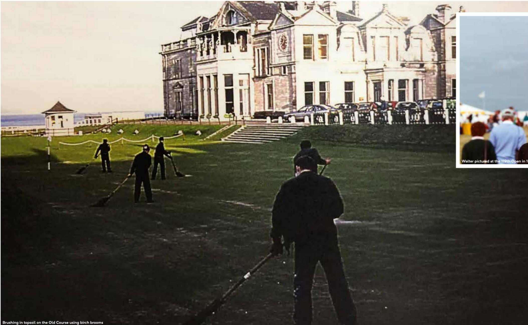
Brushing in topsoil on the Old Course using birch brooms
