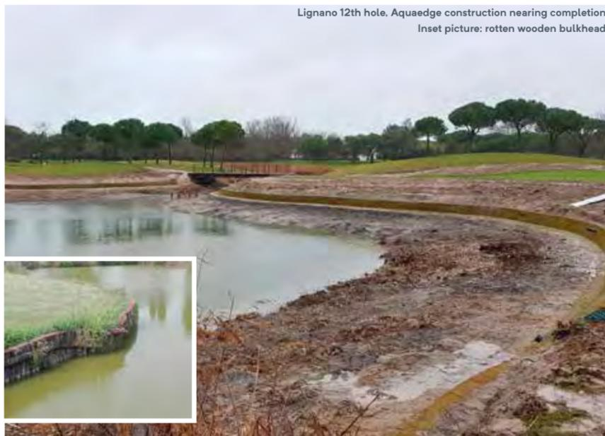
“We are currently using Aquaedge on numerous lake edges on one of our EGD projects in mainland Europe. The Aquaedge product has provided not only a structural solution to previous eroding lake edges, but has satisfied the aesthetic design intent by still providing the desired clean grass edge down to water level. EGD and the client have been delighted with how the product is performing.” — Dave Sampson, Designer, European Golf Design
