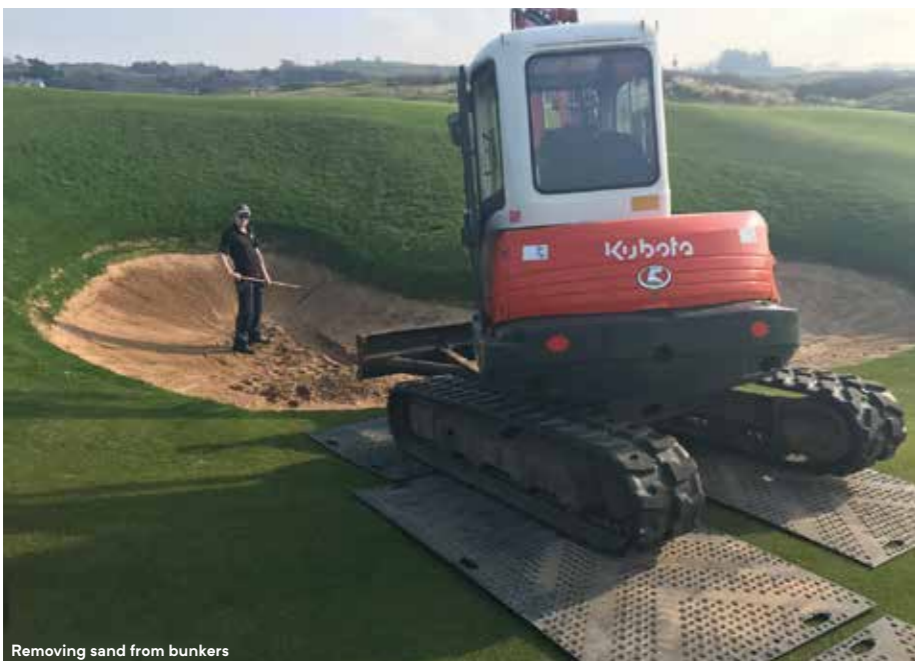
Removing sand from bunkers
