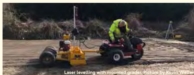
Laser levelling with mounted grader. Picture by Kevin Weller
