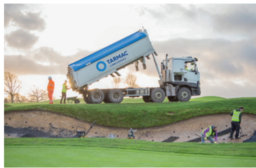
Installing Tarmac's Topsport lining
