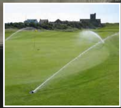
Background: Good Sprinkler Coverage Top: Poor Sprinkler Coverage Bottom: Turfgrass too long affecting correct operation
