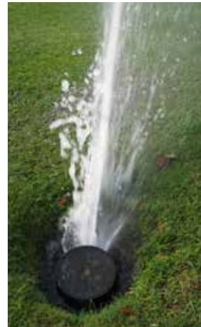
Top: Damage to cables from vermin Bottom left: Sprinkler too deep affecting correct operation
