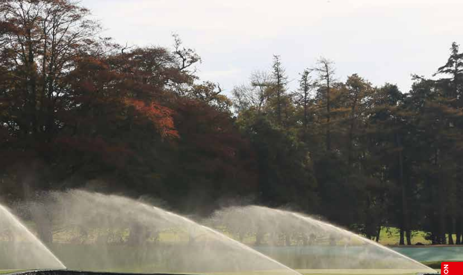
Background: Good Sprinkler Coverage Top: Poor Sprinkler Coverage Bottom: Turfgrass too long affecting correct operation
