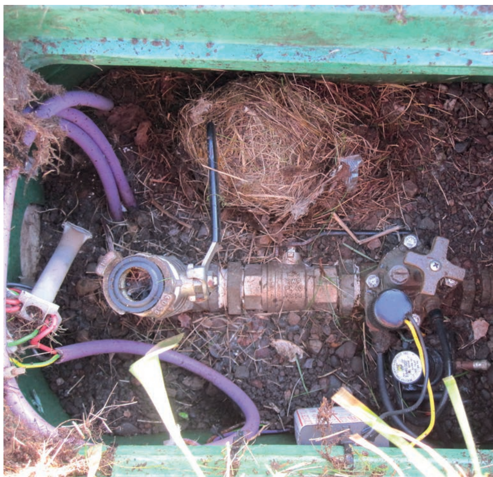
Fauna-Vermin in Valve Boxes will Damage Cables and should be removed
