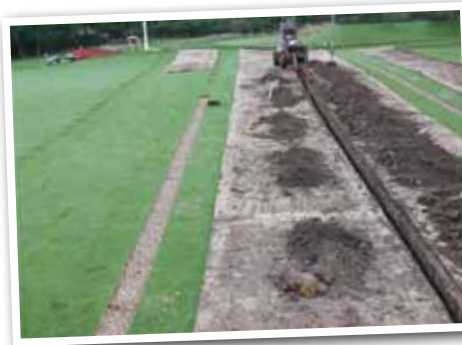
TOP RIGHT: PCD installation with narrow sand curtain RIGHT: Drainage Triangle above PCD immediate post install INSET ABOVE: Old method of trench install
